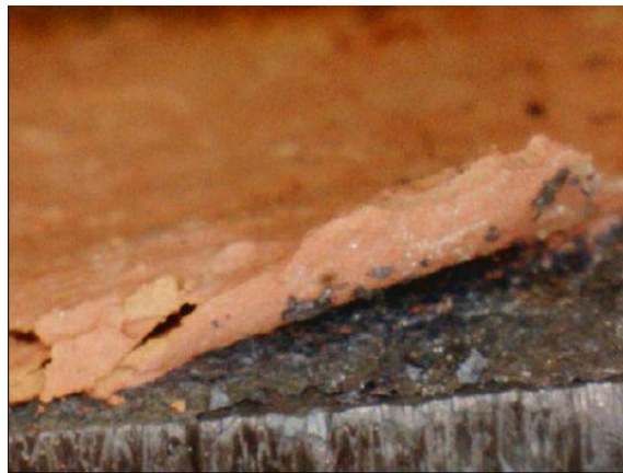
Source: NIST. Figure D-4. Formation of a black scale between paint and steel after exposure greater than 650 °C. Paint readily spalled.
