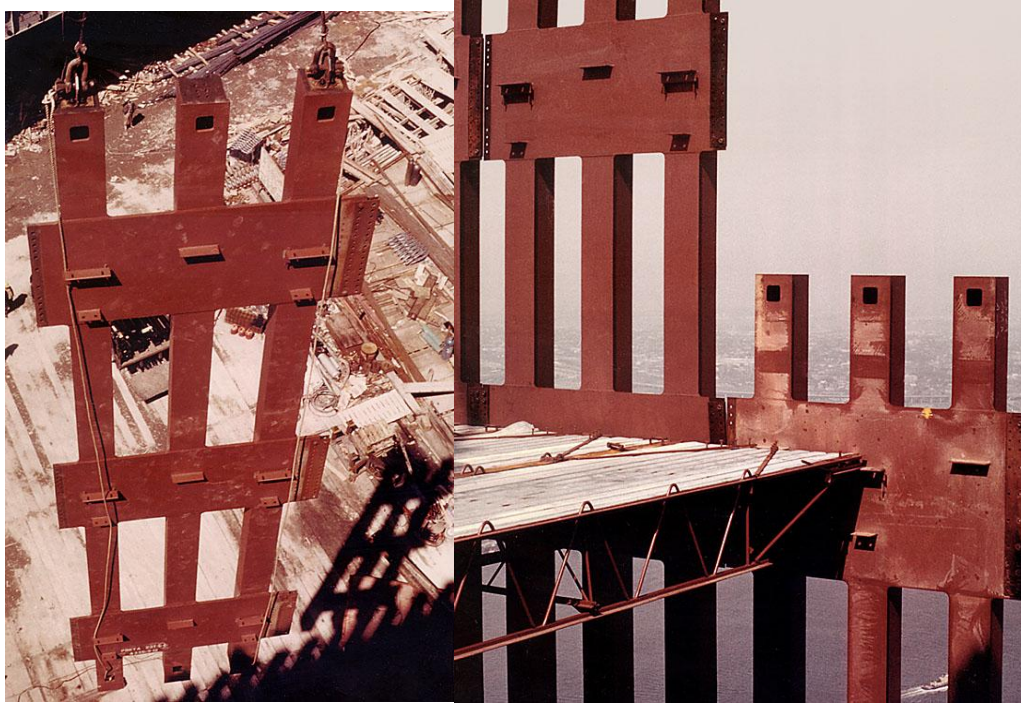
Figure 2. Perimeter columns in WTC towers. From NIST.
